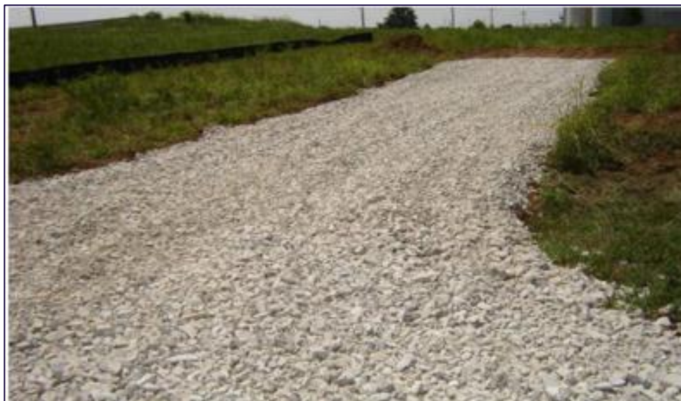
Figure 8.1: Temporary access track
